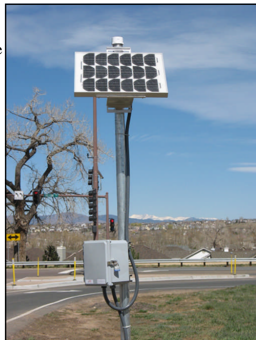
WFL-DC Remote unit with solar power at flow sensor and MV site
